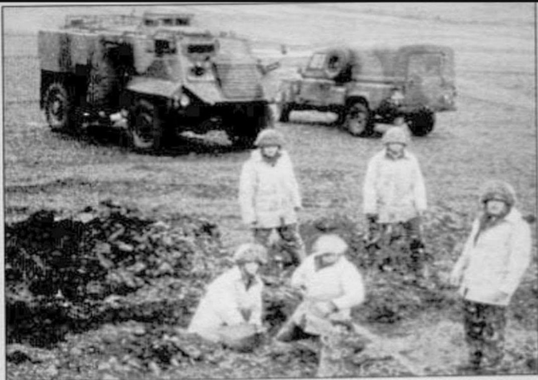
Some of the sappers at work in one of the trenches excavated at Scatsta. Photo: Gordon Stove
